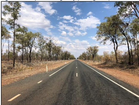
Figure 3.1: Capricorn Highway (Facing East)
